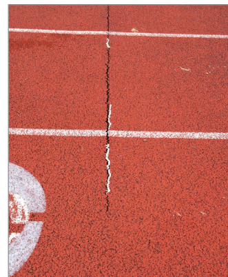
The above photo shows the cracked surface of the track, which is over 11
